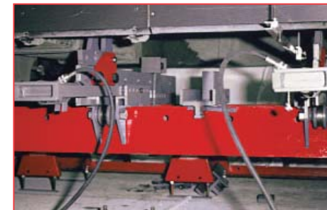
THIS IS A "DOUBLE PUSH" SET UP USED TO CORRECT A SIDE SWAY CONDITION.
